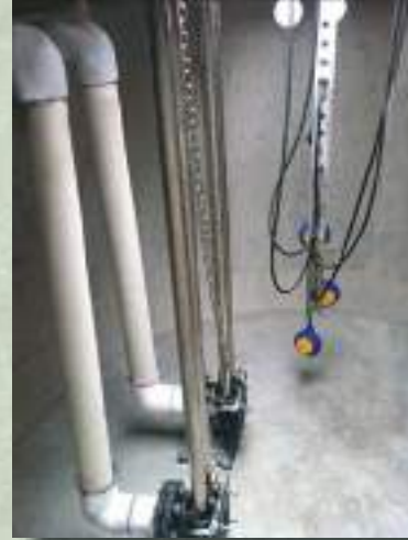
Pipework, Rail Kit and Floats installed
