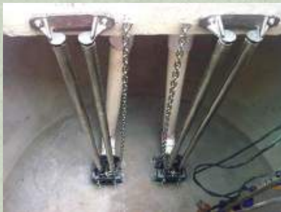
All stainless steel rails, bolts, lifting chains and float assembly
