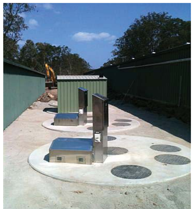
2 x CABS Tanks installed at the Lake Moogerah Ski Club
